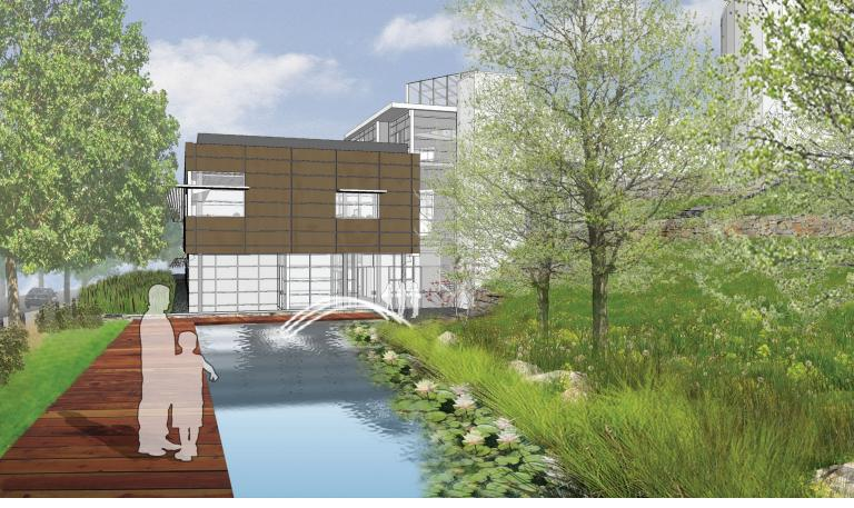
The CSL's lagoon system captures stormwater runoff from throughout the site and replicates the natural water treatment process that occurs in wetlands and marshes.
